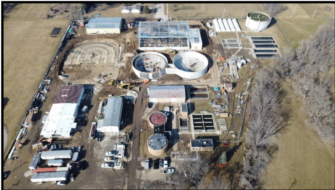
(Waste Water Treatment Plant Expansion Project)
