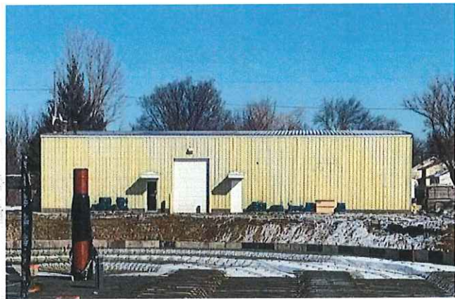
Existing Storage Building - WWTP
