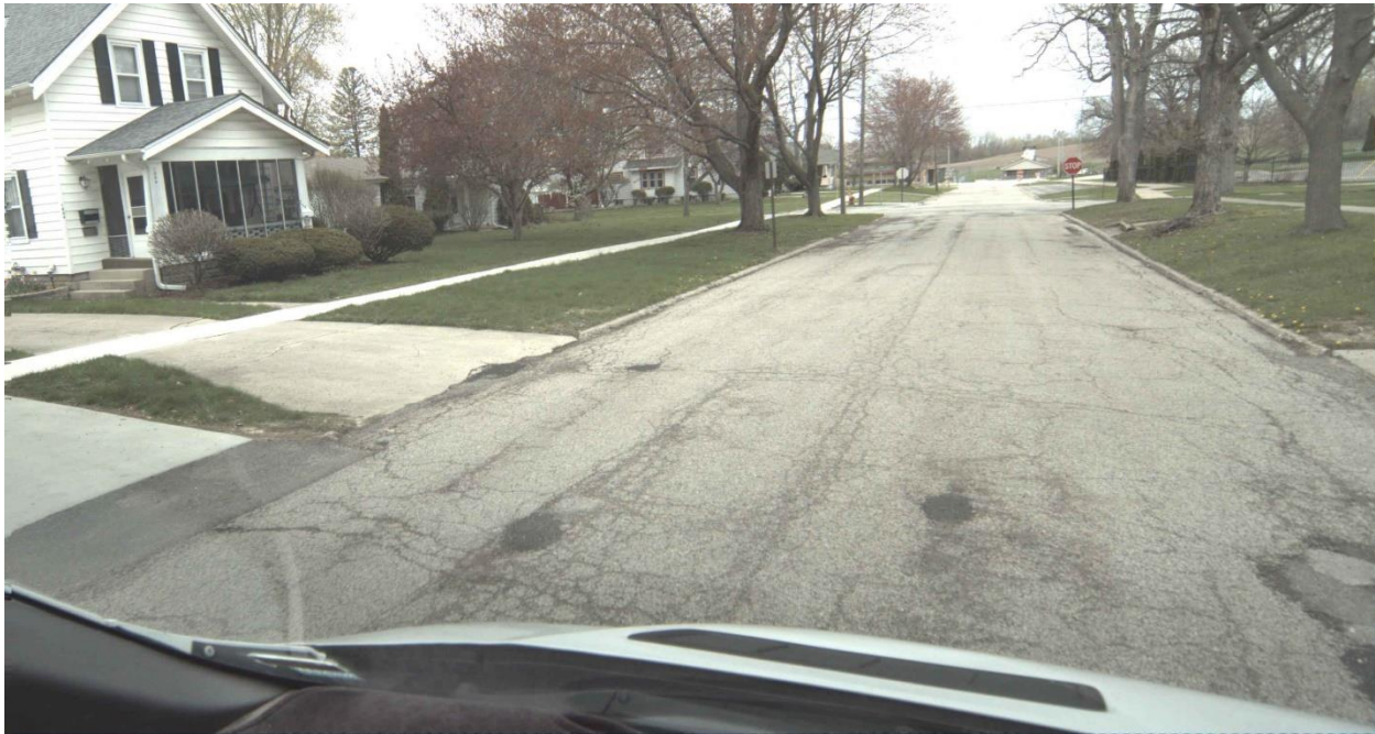
Figure 10 - Example of a Pavement Rated as Very Poor
