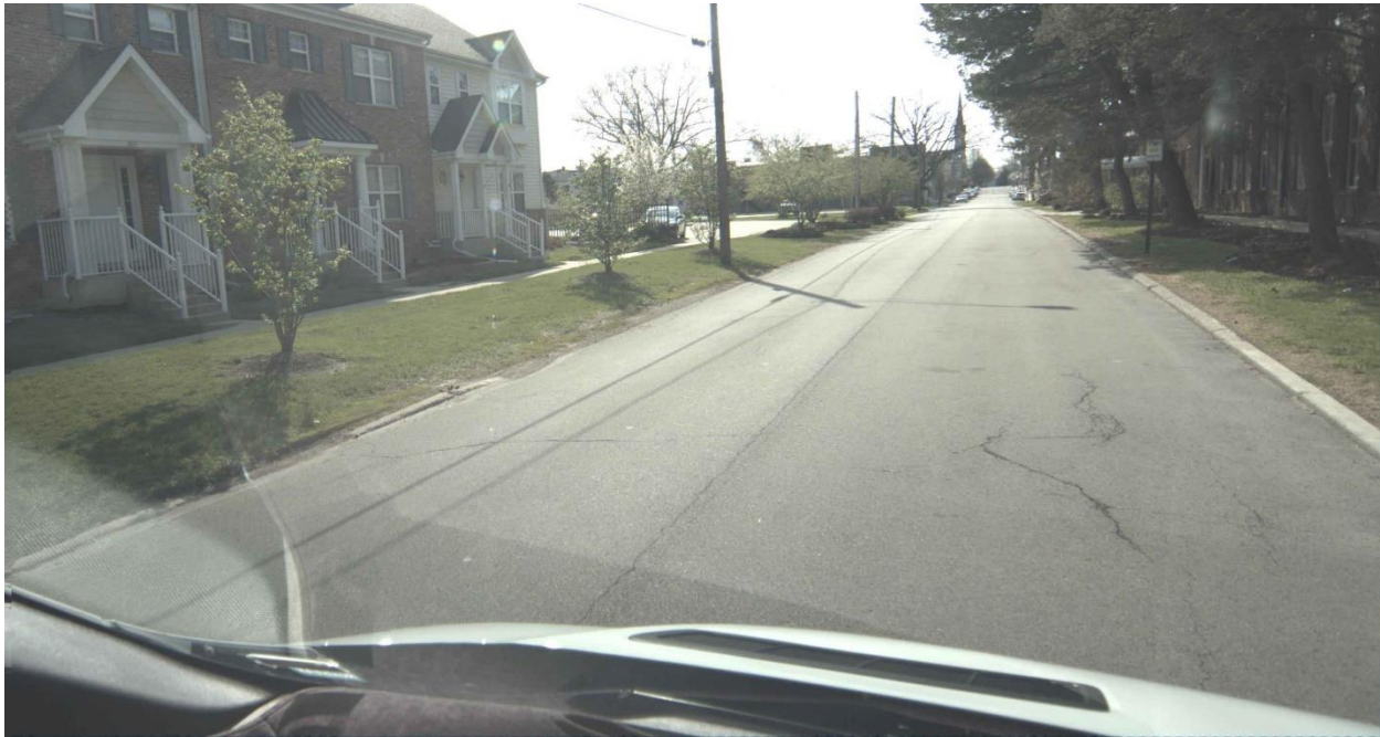
Figure 13 - Example of a Pavement Rated as Satisfactory
