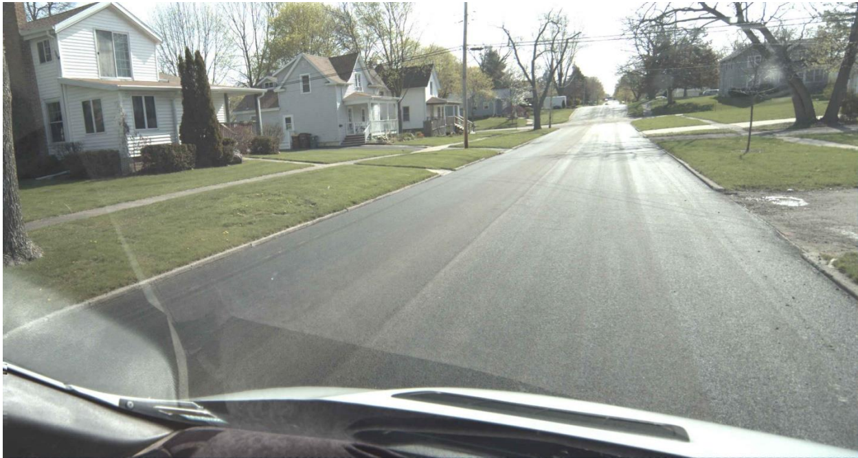
Figure 14 - Example of a Pavement Rated as Good
